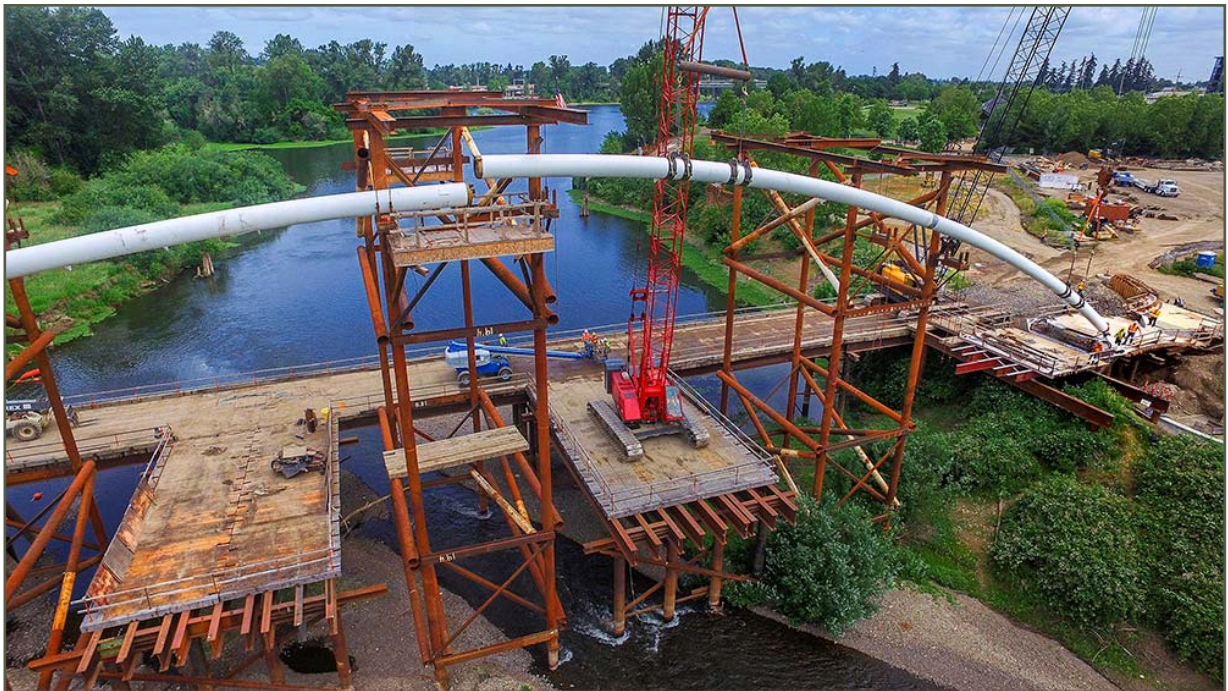
Arches being installed on the Peter Courtney Minto Island Bridge—Photo courtesy of Ron Cooper
