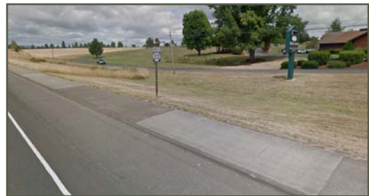
Portions of the damaged asphalt have been replaced.
