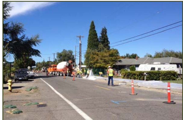
Auburn Road-pouring sidewalk
