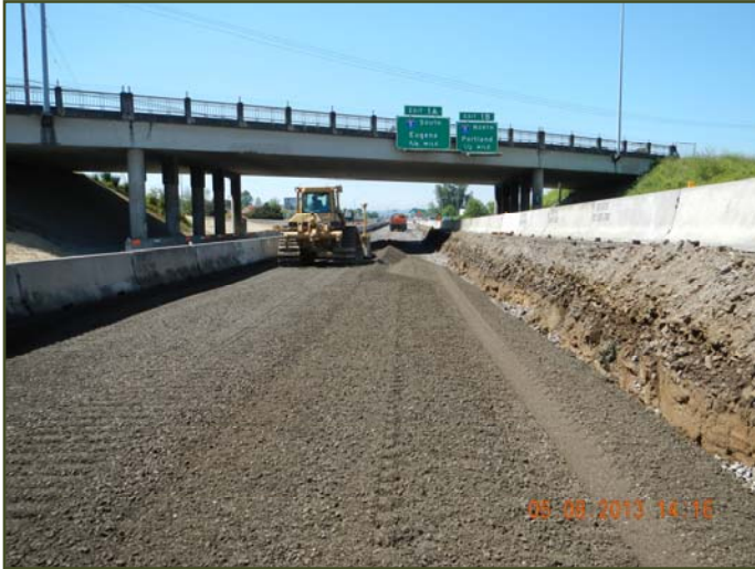
OR 22E at the Lancaster Drive overcrossing- Digging down to increase the vertical clearance at the structure.
