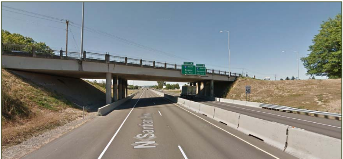
OR 22E at the Lancaster Drive overcrossing-Vertical clearance increased.
