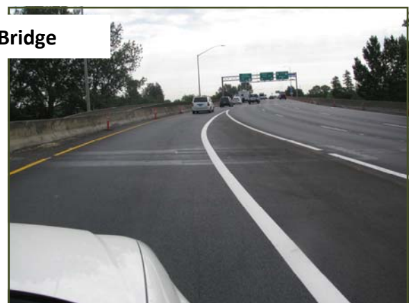
After—Repaired joint and new pavement.
